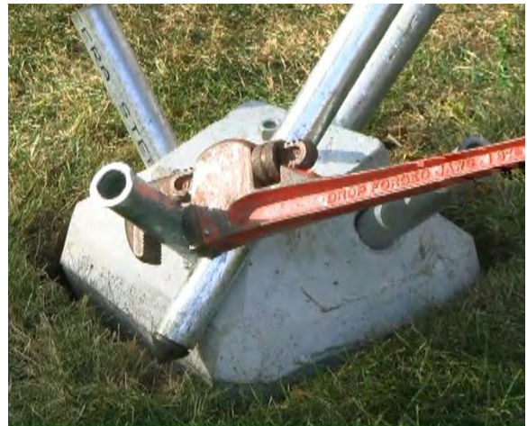
Figure 6. Jacking Method for Pin Removal
