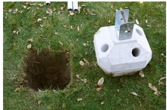
Figure 3. Tapered Hole for Concrete Head
