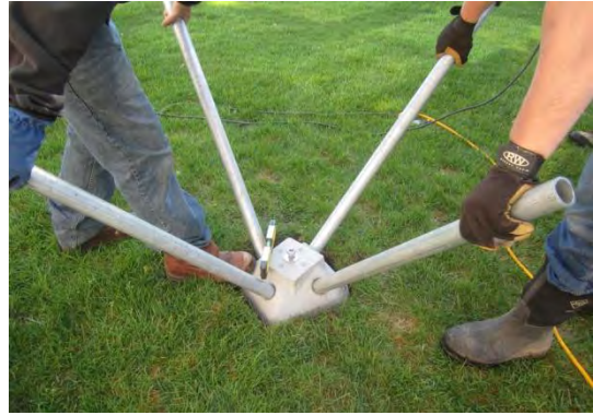
Figure 4. Setting Pins and Leveling Pier
