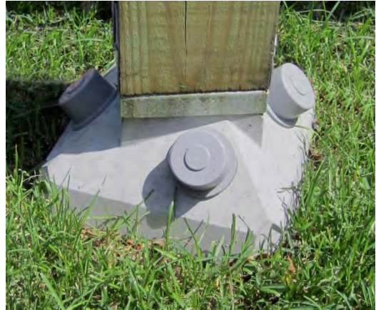
Figure 7. Completed Installation with Pin Caps
