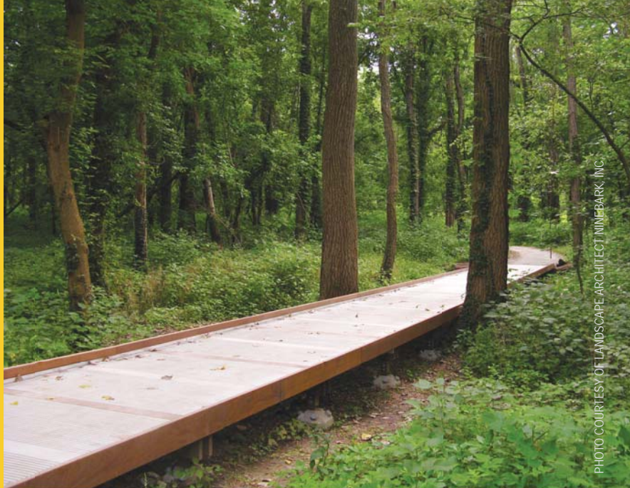
Diamond Pier foundations made possible the construction of this walkway with minimal site disturbance in this historic forest. Virginia B. Fairbanks Art & Nature Park – Indianapolis Museum of Art.
